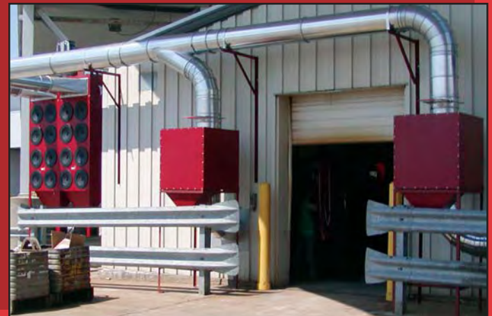
RP8-2 with spark arrestors collects laser smoke.
