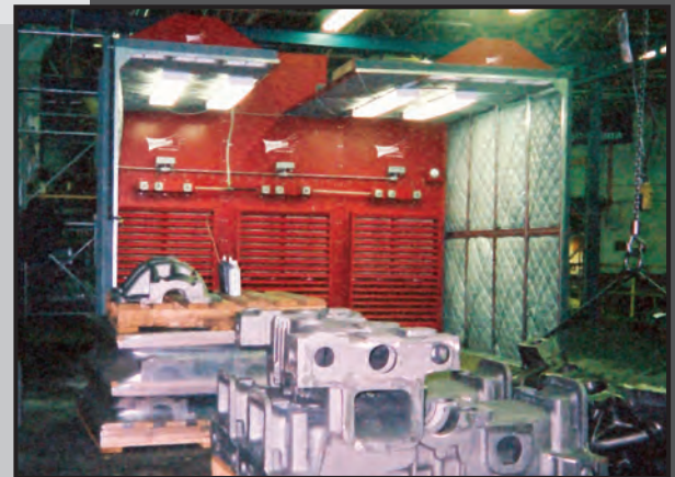
Clean Air Booth with Crane Slot
