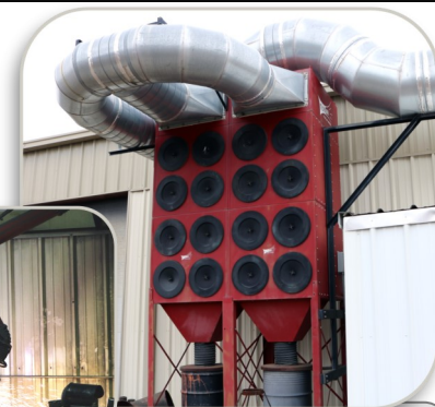
Source Capture Arms ducted to central system located outdoors returns clean, heated/cooled air to facility.
