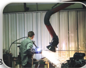
Source Capture Arms ducted to central system located outdoors returns clean, heated/cooled air to facility.
