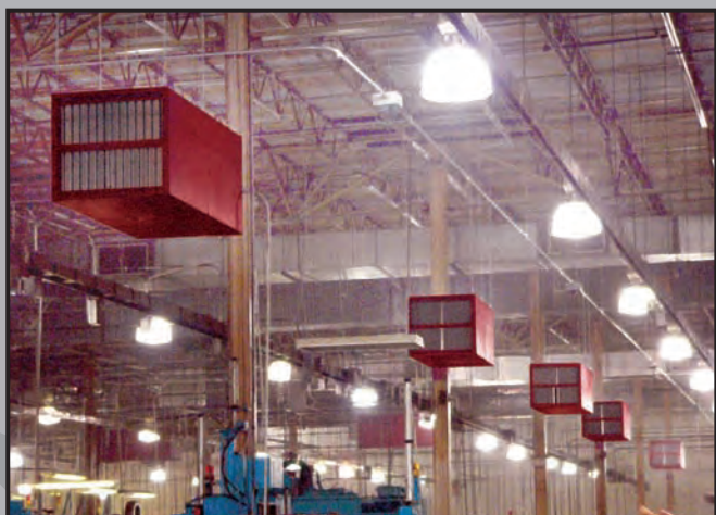
Horizontal 6000 cfm Mist collectors mounted in race-track Configuration for ambient capture of mist.
