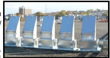
Roof Penetrations for Explos. Vents
