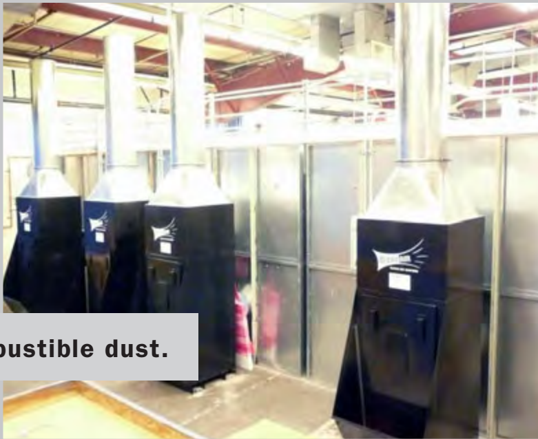
Combination of Booth Enclosures and Downdraft Tables ducted to combustible dust operations with titanium and aluminum.
