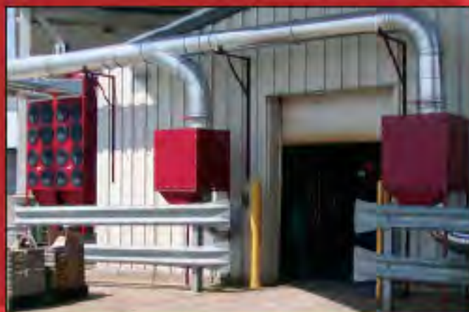
RPB-2 with spark arrestors collects laser smoke.
