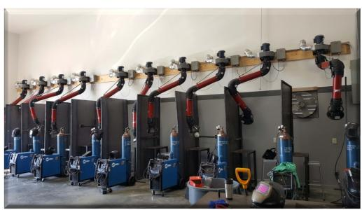
have some type of extraction in their work area. In order to make this possible the layout was changed to a combination of source capture arms exhausted outdoors and the XA23 Downdraft Tables.
