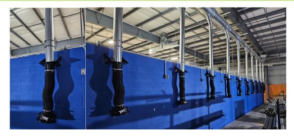
Micro Air is excited to share the first large install of the 6 inch Telescopic SCTA arms. This is new construction going into a college to capture weld smoke from the work stations powered by a large RP12-3 & 100 HP motor. This project is undergoing.....But what a great example of our distribution network providing a solution!
